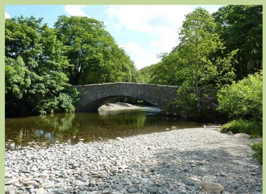
Forge Bridge access area
